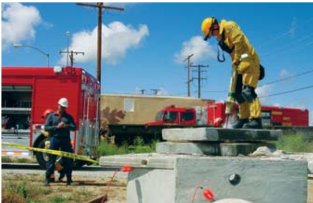
The LACoFD's Regional USAR Task Force is tested on search cutting and breaching operations during one of several simulated collapses.
