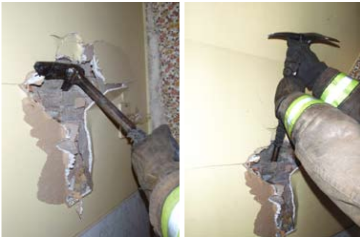
For opening drywall and plaster walls, I swing the awl into the wall and push up, creating a hole. I then drop the forked end in the hole about a foot and keep ripping the awl away a little at a time.
