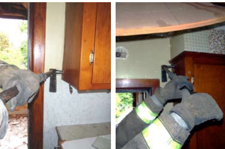
After driving the awl of the Halligan into the cabinet you can push down or pull toward you to pop the cabinets from their mounting.
