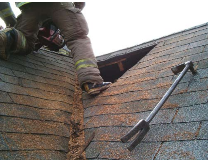
Planting the awl of your tool into a peaked roof surface will give you an extra step should you need it.
